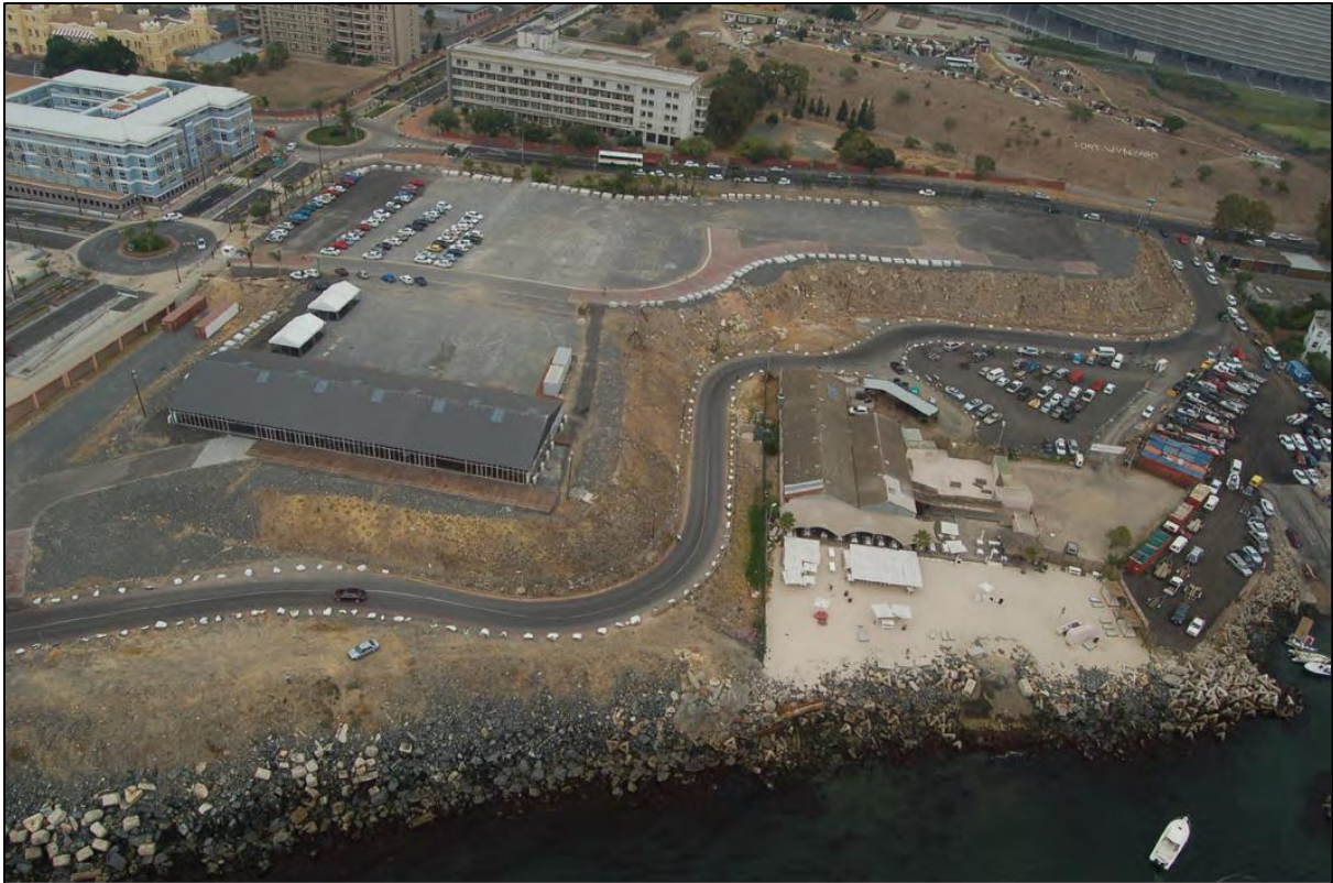
Plate 2: Aerial view of a portion of the land reclamation project site looking south and showing the deep fill between Jetty Street and Beach Road, and the existing rock revetment along the coast (After: Baumann 2015).
