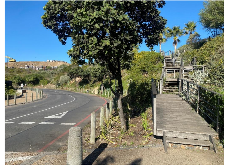
Photograph 3-9: Pedestrian walkway next to Haul Road (left) and stairway to the parking structure (right)
