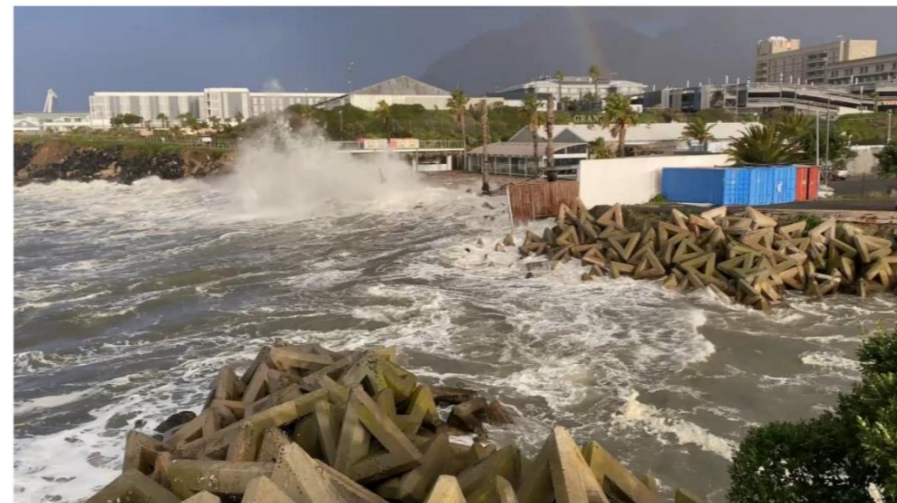
Photograph 4-5: Overtopping in front of Grand Café and Beach on 13 July 2020 (exact time unknown). Photo credit: Anton Holtzhausen (PRDW, 2023)
