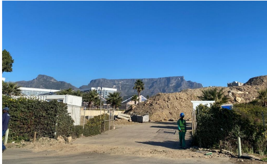
Photograph 4-1: The previous Lookout Centre is currently utilised as a construction storage area
